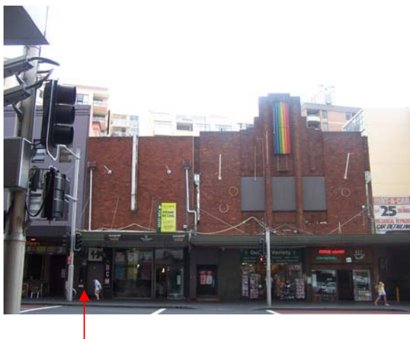
Figure 1: Entry to premises. Nightclub with residential apartment blocks behind.
